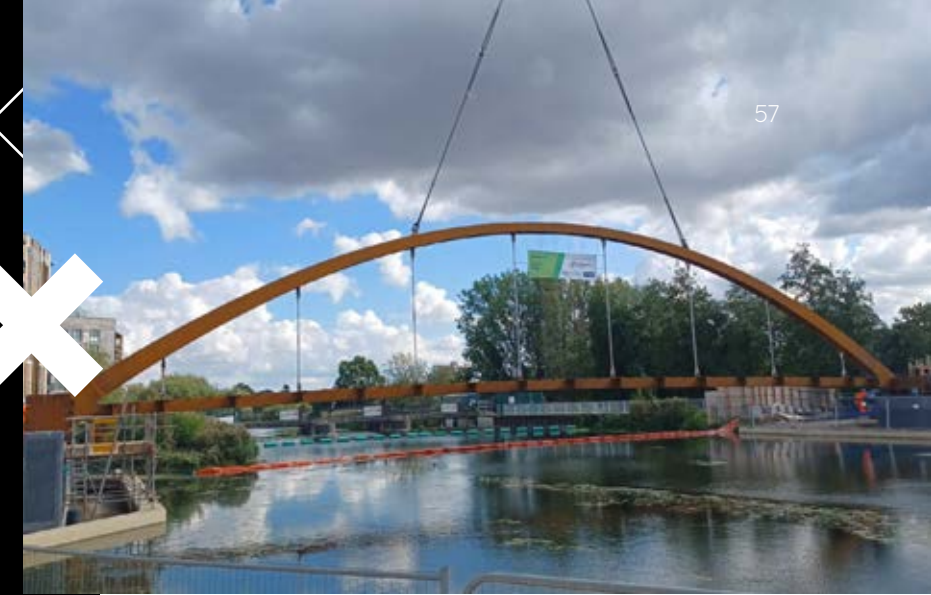
Image: Bow Bridge Road © Chelmsford City Council
